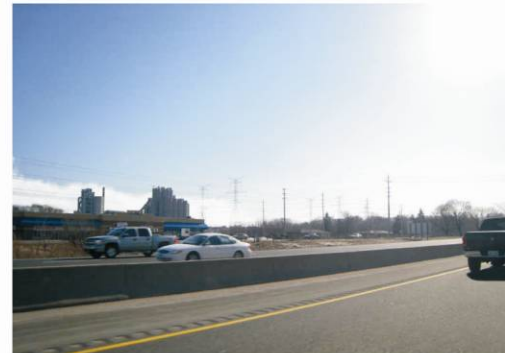
Mechanical Draft Cooling Towers Highway 401 Westbound, Facing South-West (No-Foliage)
