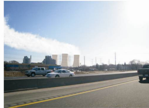
Natural Draft Cooling Towers Highway 401 Westbound, Facing South-West (No-Foliage)
