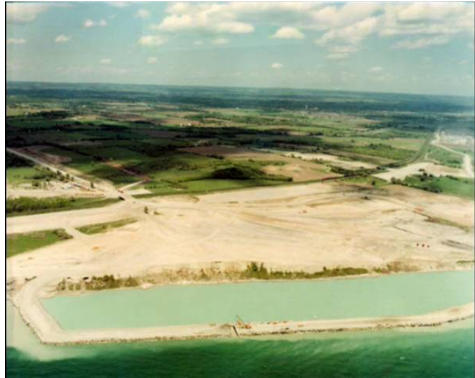
Cofferdam Construction for DNGS
