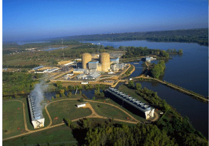
Mechanical Draft Cooling Towers at Prairie Island, Minnesota (Nuclear Tourist Web Site 2008)
