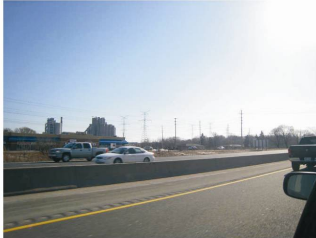
Highway 401 traveling Westbound, north of the DN Site Facing South-West (No-Foliage)
