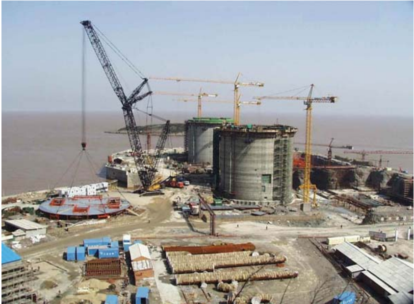
Construction of CANDU-6 Nuclear Power Plant at Qinshan, China using Liebherr LR1600/175- Very Heavy Lift Crane (Rixin and Petrunik 2003)
